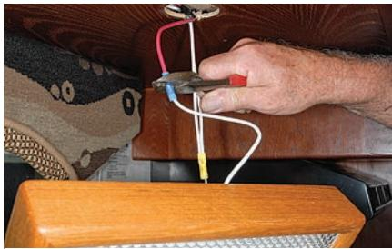
(Above left) The Alpenglow installation requires connection of 12-volt DC positive and negative wires. Don't rely on color coding; check polarity of power leads before butt connecting wires. (Above right) Alpenglow's Caribbean Reading Light has a metal on/off rocker switch and rheostat to adjust intensity of the light, a feature that gives users better control for reading in bed.
